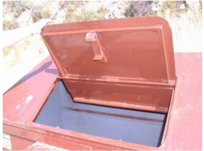
Figure 7—A counterbalanced door allows easy lifting.
