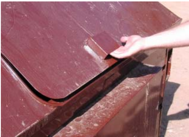
Figure 6—Bearproof latch on counterbalanced door. Note bear claw guard all around.
